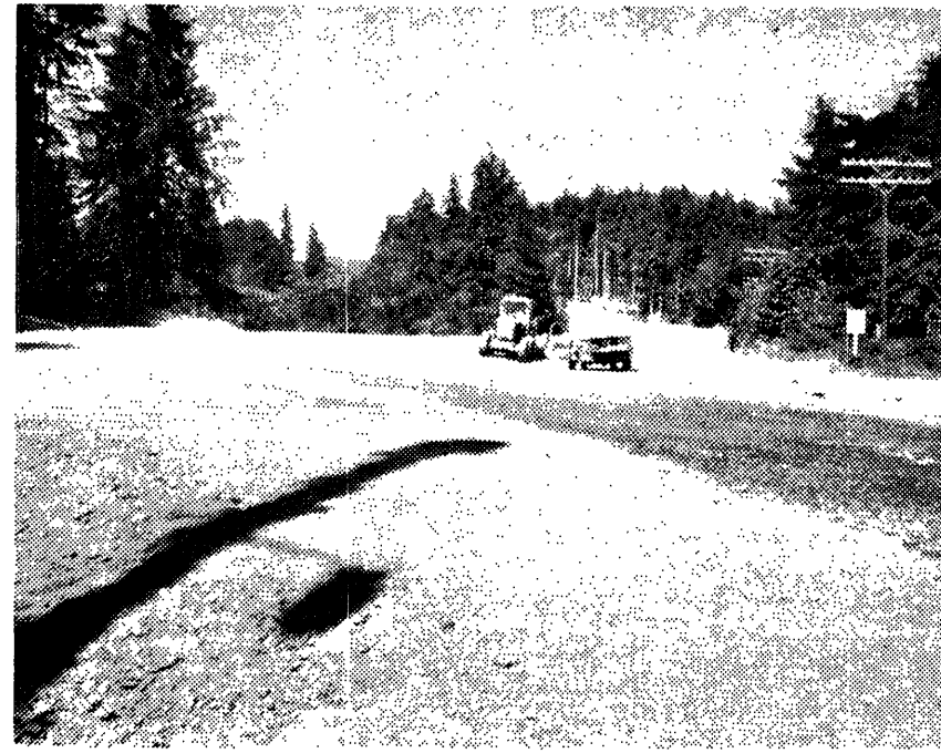
BURNT MOUNTAIN ROAD CONSTRUCTION LOOKING FROM SAPHO JUNCTION.
