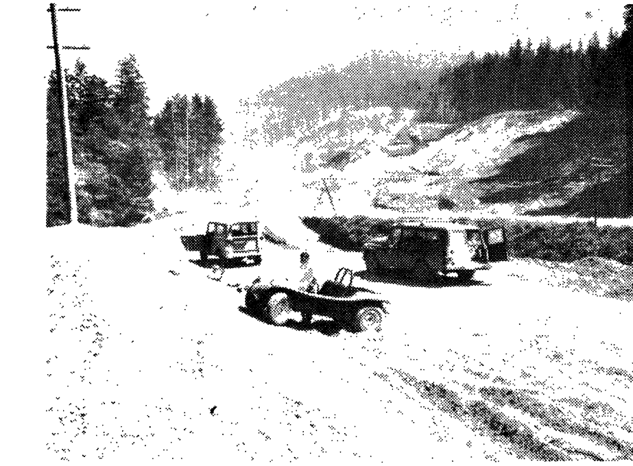
FILL IN FOREGROUND AND CUT NECESSARY IN CONSTRUCTION NEAR SEKIU ON HIGHWAY 112.
